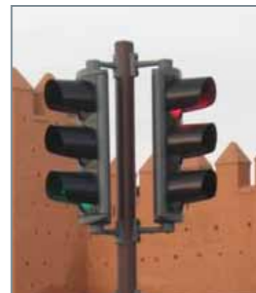
Conventional two-point-fixation with bracket arms
